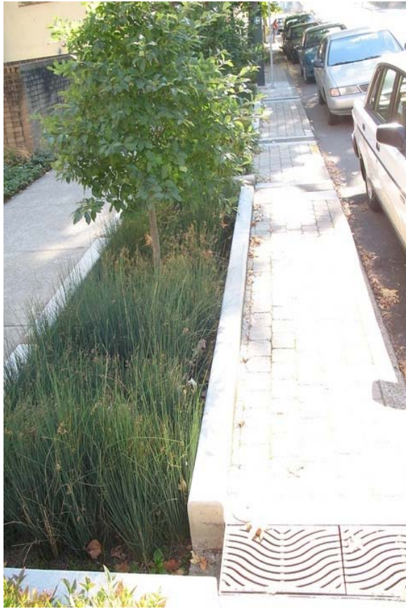
Natural drainage system in Portland. (Bioswale style)
