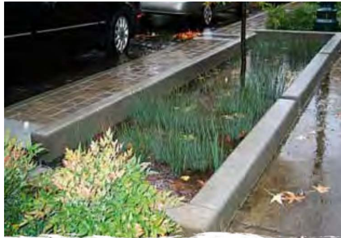
Bioretention areas filter polluted road run-off, provide urban wildlife habitat and reduce local flooding
