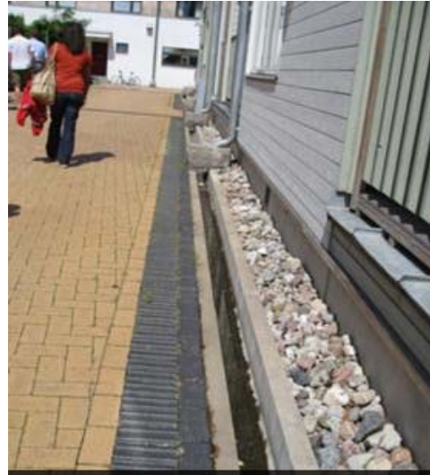
Rainwater managed above ground by a relatively simple network of channels, retention basins, ponds & waterfalls.
