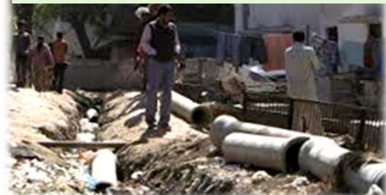
Broken Sewerage Pipes
