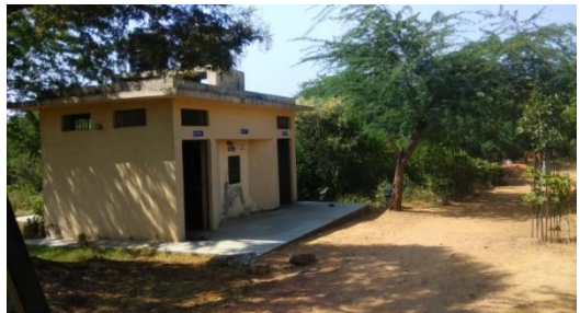
PUBLIC TOILETS (5 NOS.) SPOT SIGNAGES: 1 EACH = 5
