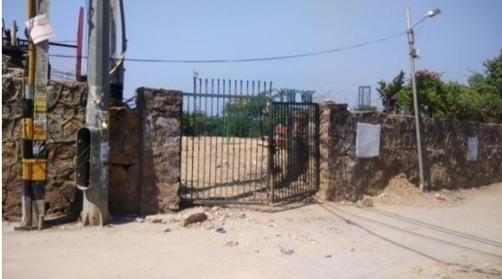
GATE NEAR KISHAN GARH (OPEN GYM)
